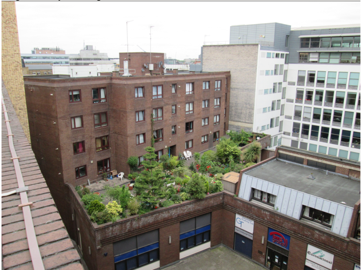
Image 4: Rear courtyard facing elevation of 10 Epworth Street with first floor terrace garden.
